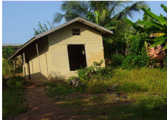
Photo 8.3: Agrochemical Storage Room under Construction
