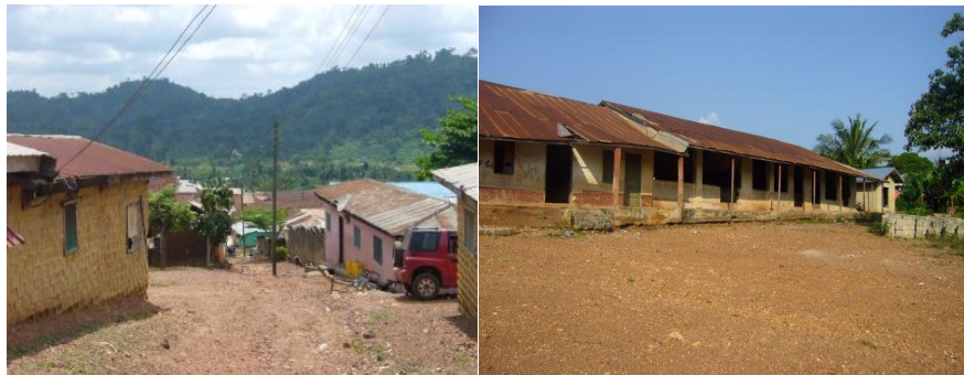
Photo 4.1: Aponapon Community Housing and School Structure
