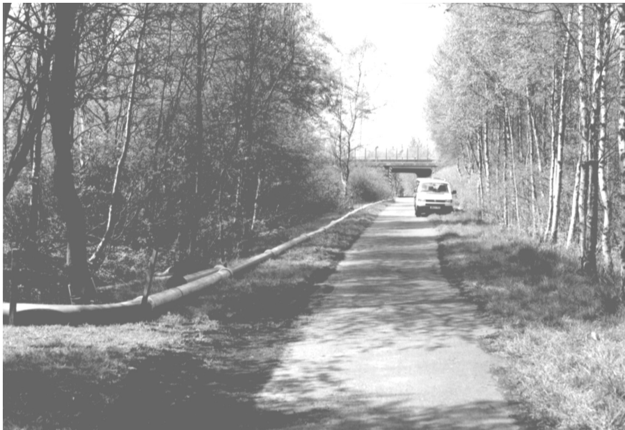
Figure 3.29: Photo from site WD with a view in western direction along the asphalt track. At the left is the outlet tube of the pump in B1_{WD} . T1_{WD} is right beside the car that was later used for a loading test. In background is a bridge of the freeway.
