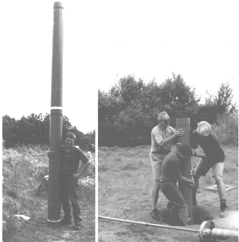
Figure A.2: Installation of the casing, T1 OE . In the front of the right photo the second, manually operated drilling tool (Eijkelkamp, 1998) is depicted.
