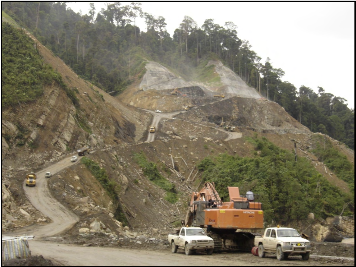
Picture 3: Work in progress in Bakun in October 2004
