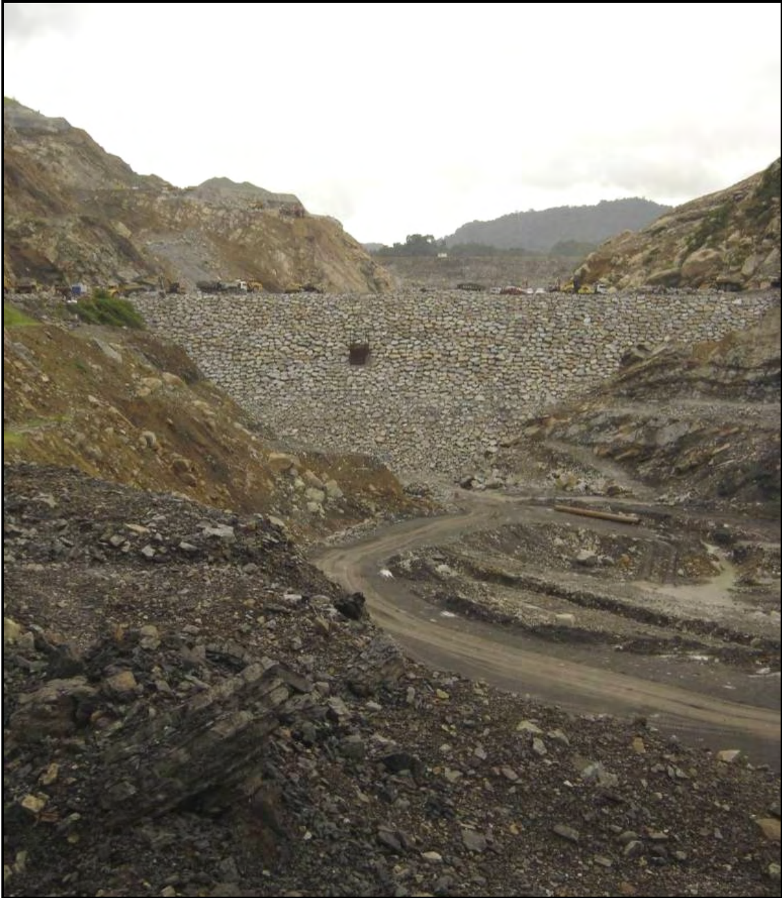
Picture 2: Bakun dam under construction in October 2004
