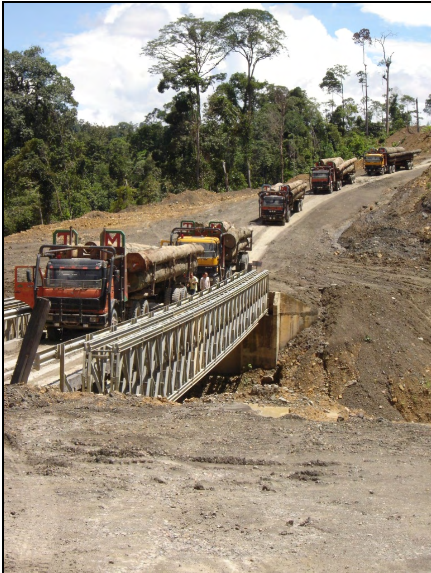
Picture 4: Temporary bridge on gravel road used by logging trucks
