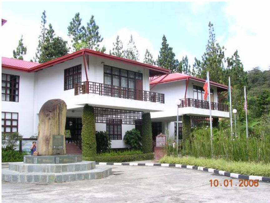
Figure 4.2 Sabah Parks administration building in Kinabalu Park. The World Heritage Site citations are inscribed on the sandstone monument in front of the building.
