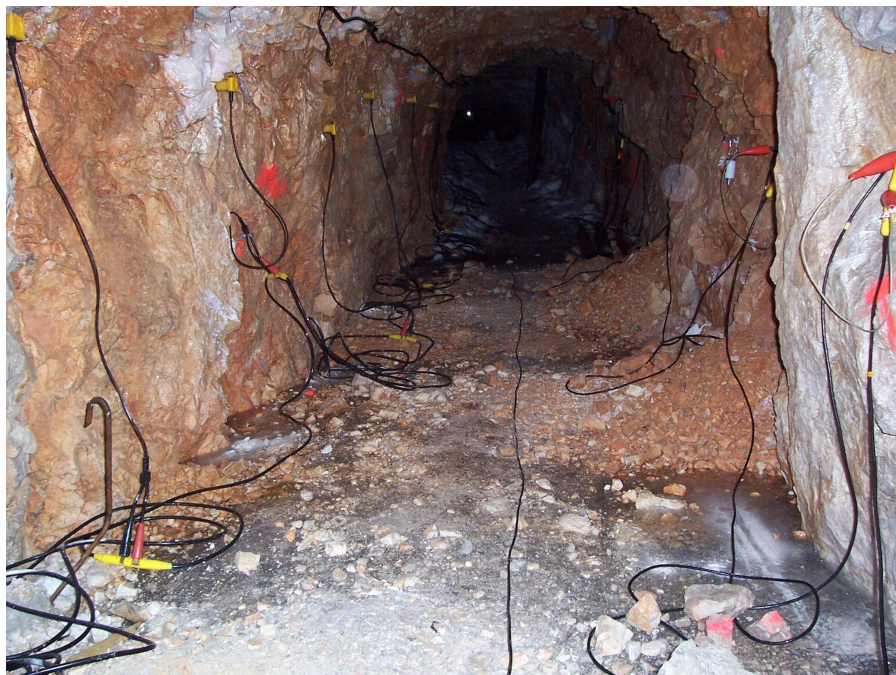
Fig. 41: Geophysical instrumentation in the Kammstollen gallery 25 m from the North Face at 2800 m a.s.l.. Permafrost is evidenced by perennial ice on the floor; the picture shows electrodes and a temperature logger on the right side.
