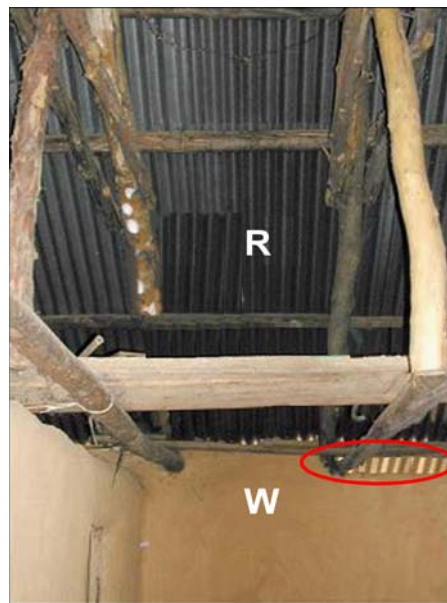
Overhanging roof (R); Wall (W) ; Eaves (circled in red)
