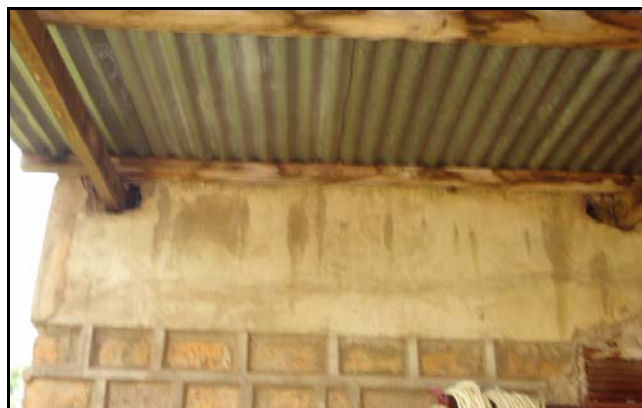
Figure 2.2 Uncovered ventilation holes
