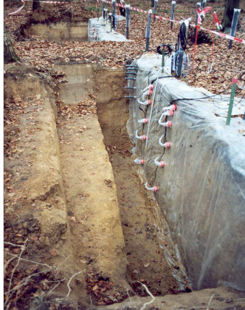
Fig. 2.4: View on trenches 2 and 3 after installation of instrumentation.
