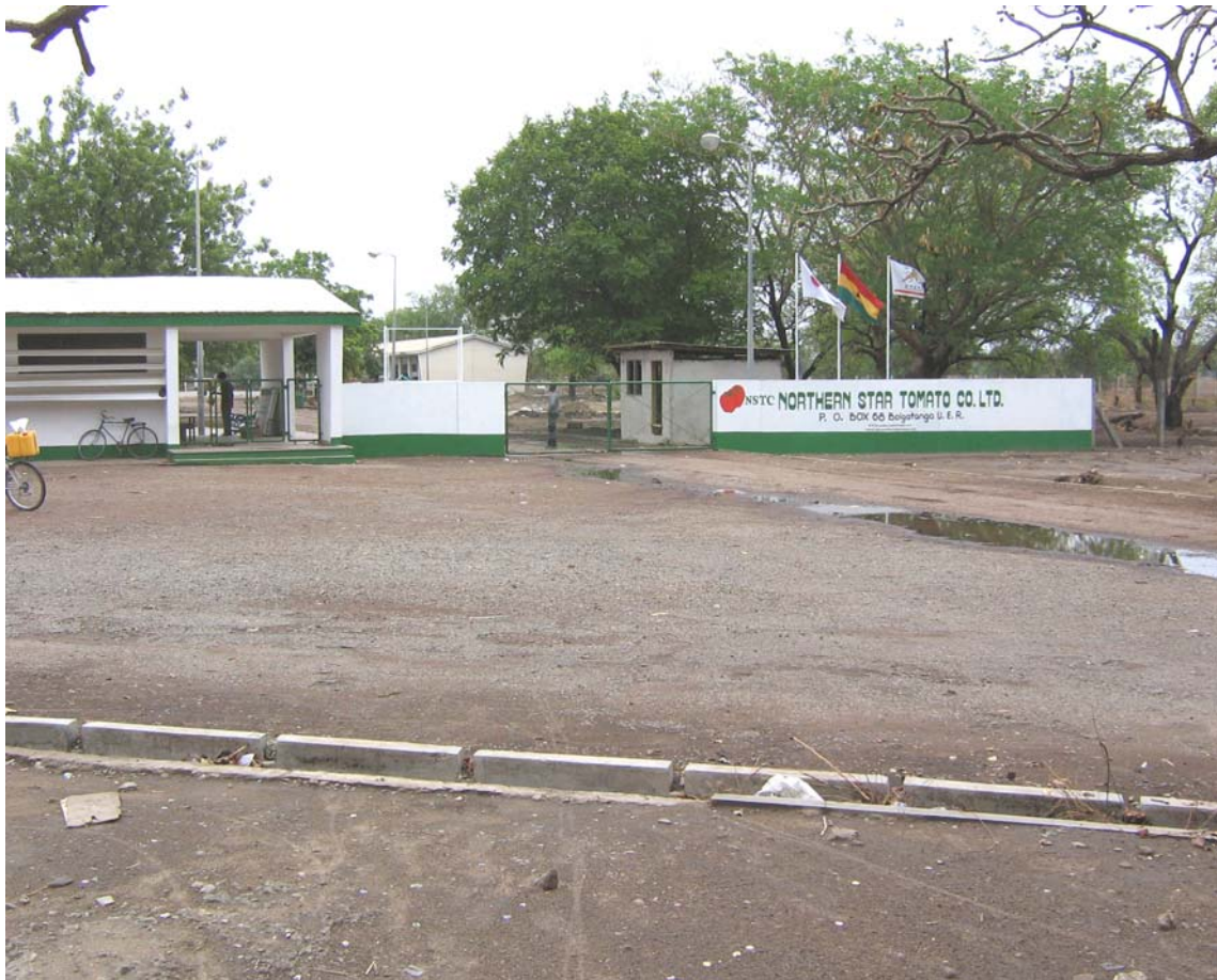
Photo V.2: Entrance to the tomato canning factory in Pwalugu
