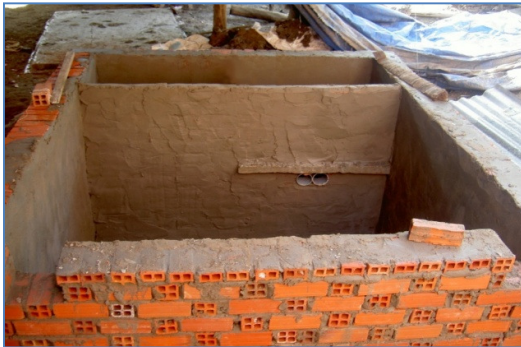
Figure 1.5 | Newly built septic tank.
