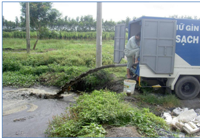
Figure 2.6 | Septage is discharged into a dump located in Hau Giang province.
