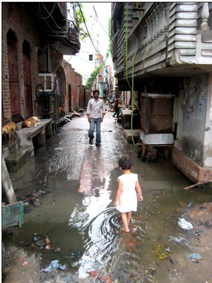
Photo 20: Problems in brick streets. Especially children are exposed to waste water when drains overflow in the rainy season. (Photo: A. Zimmer, August 16, 2009)
