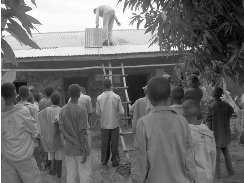
Fig. 5.2: A solar home system being installed
