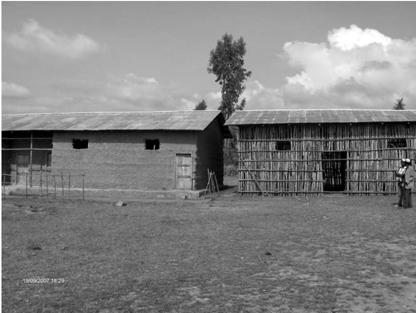
Fig. 6.2: Additional classrooms constructed fully by the community
