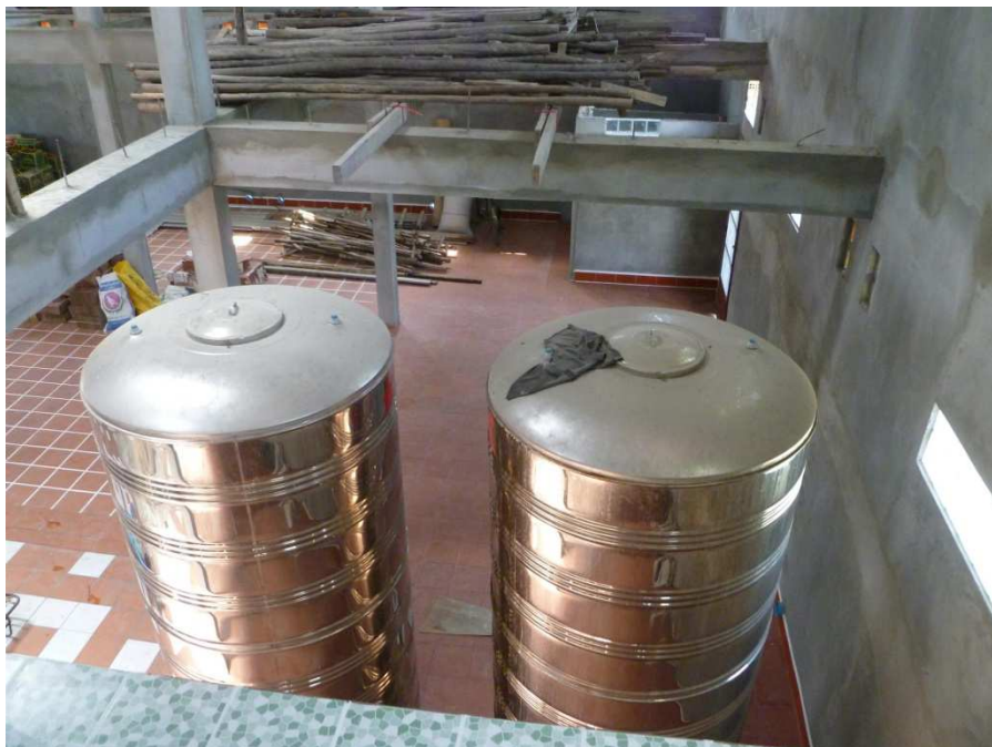
Figure 5.9 Construction of Khmer Natural Enterprises new palm manufacturing facility
