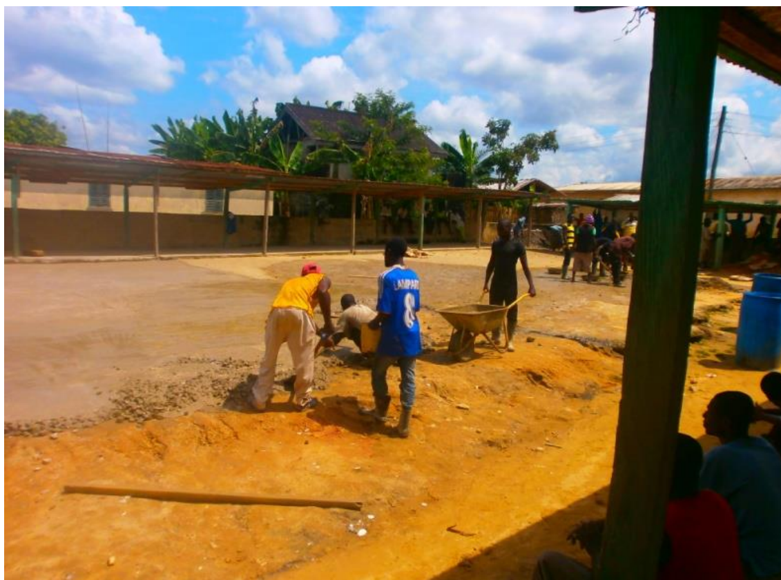
Figure 4.9: Communal labour in the construction of a community centre for Akutuase
