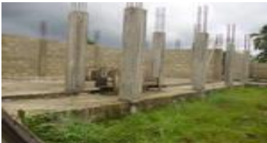
Figure 4.4: Daboase new market under construction
