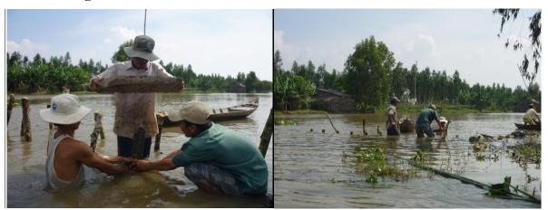
Picture 5-10. Dyke repairs before pumping (Huynh Linh 2011).
