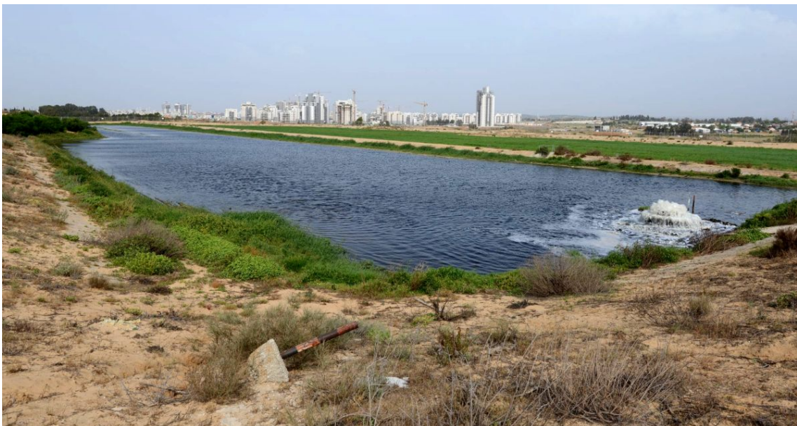
Figure 2.1: Picture of an infiltration pond from the Shafdan site in Israel (see Chapter 5) as an example for the MAR technique soil aquifer treatment (SAT) (Section 2.1.1). Note that the water table here above the surface does not exceed 0.5 m.
