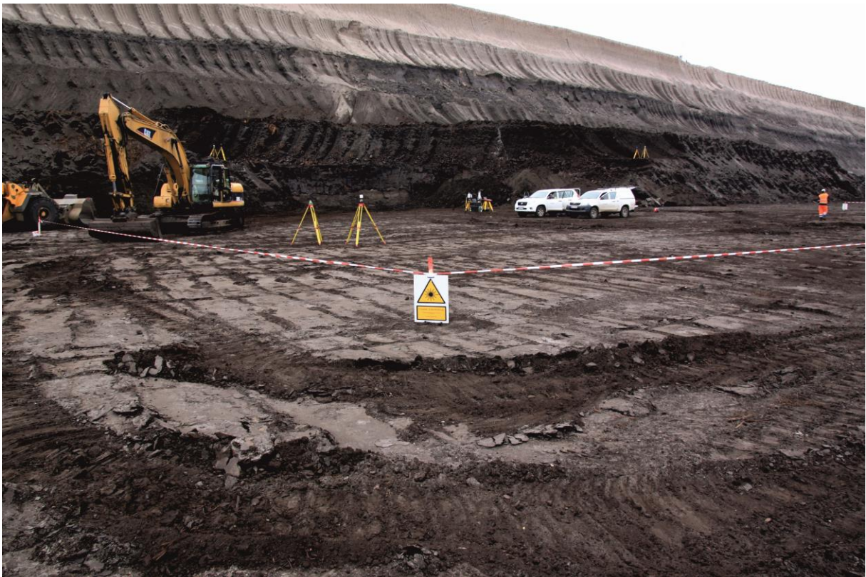
Fig. 5-1: Laser scanning of one sand body in the upper part of the Frimmersdorf Seam (11.11.2015).
