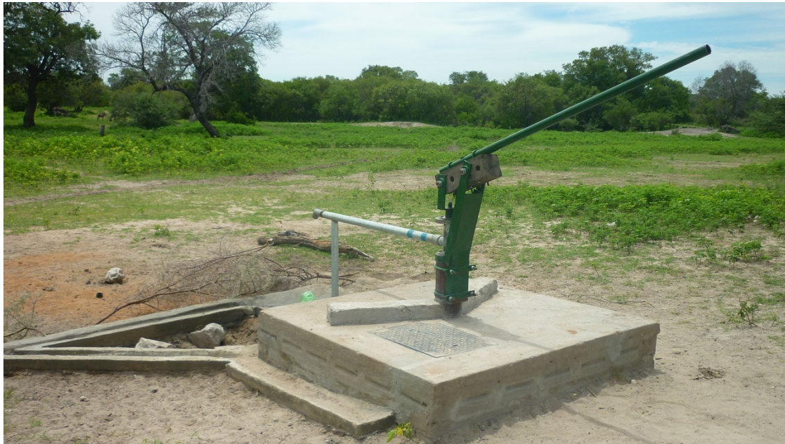
Figure 39: Improved borehole in the dense woodland of northern Namibia, east of Eenhana. The covered surface prevents contamination of the well water and provides high quality drinking water even during the dry season (Photo: Luetkemeier 2014).
