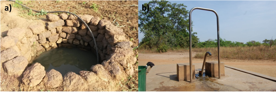
Figure 2.16: Examples of unimproved and improved water sources. (a): Open well in Burkina Faso, 2015; (b): Covered borehole with a foot-operated pump in Benin, 2013. All photos by the author.
