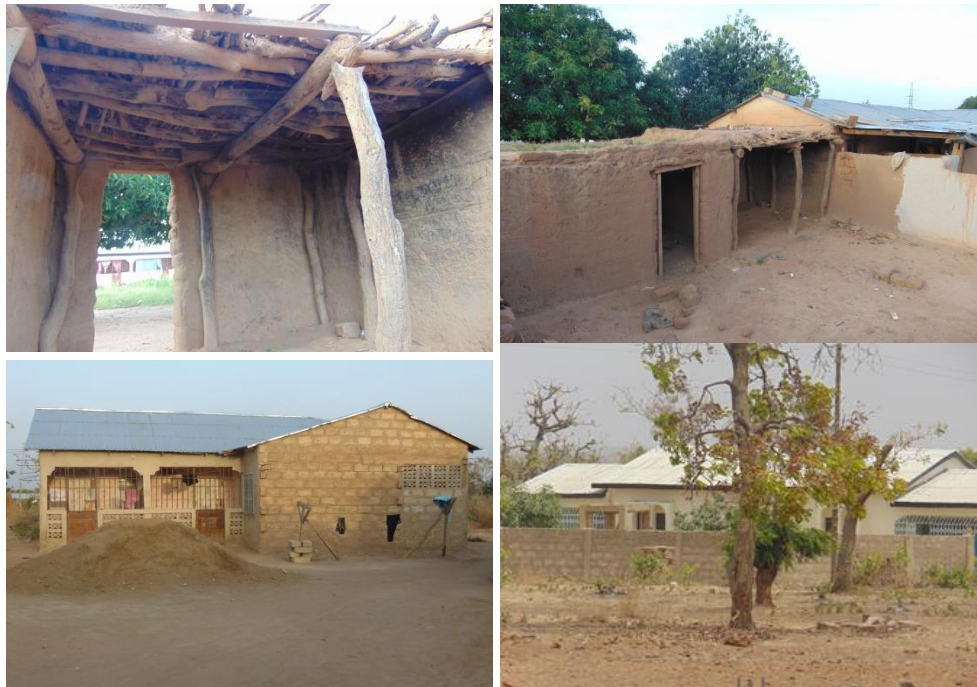
Plate 6. 4: Top: Old Traditional Mud Buildings. Bottom: New Modern Cement Block Iron-roofed Buildings in peri-urban Wa Source: Photos by Darius T. Mwingyine (2016)
