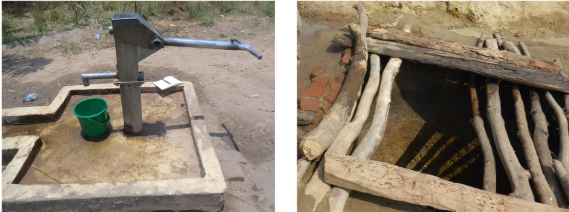
Figure 2.5 A modern and sealed pumping well in the city of Ifakara, which gathers groundwater at about 30 m depth in the left picture. The right picture shows an open well in the surroundings of Ifakara that is prone to contamination from the surface. Both wells are typical examples for water sources in the city and its surroundings (pictures taken by the author).
