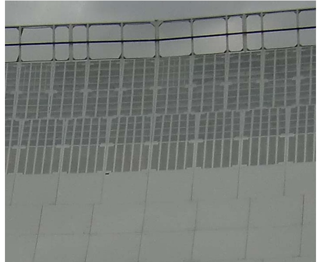
Fig. 6. Detailed picture of the reflector surface showing single panels and its perforated outer ring.
