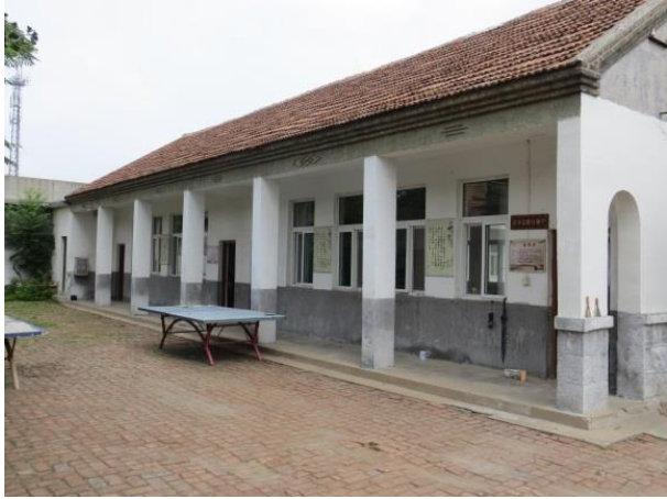
IMG. 42: Qufu academy, class room buildings on campus.
