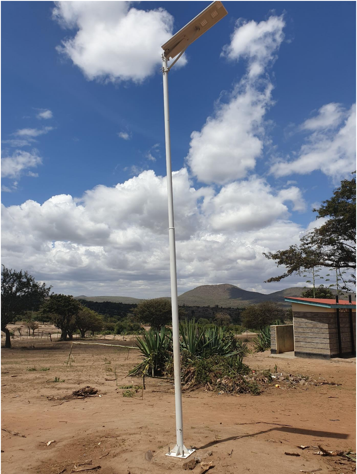
Figure 7 Solar light installed at Ilkimati Primary school in Narok county. Photo A. Ogolla 2019
