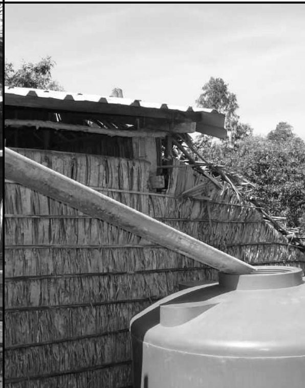
D: Sophisticated Rainwater Collection in Special Water Storage Tank
