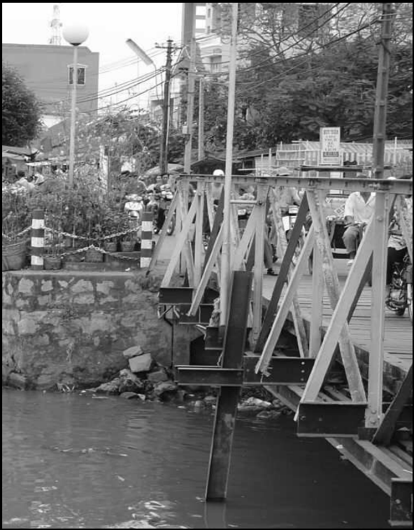
D: Modern Concrete-Steel Bridge
