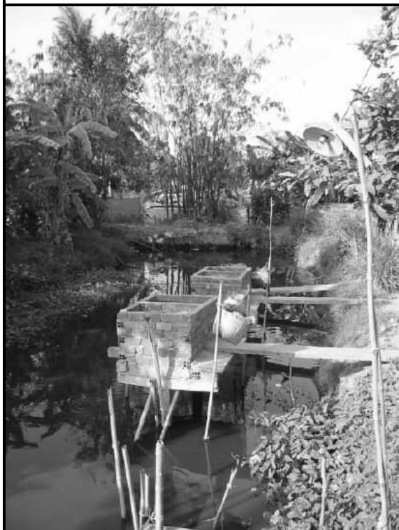
C: Sophisticated Brick Fishpond-Latrine including Electric Illumination
