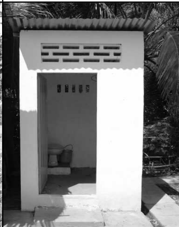
D: Modern Latrine (septic or DVC)
