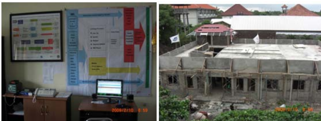
Figure 45: Temporary (left) and new EOC (right) under construction in Bali
