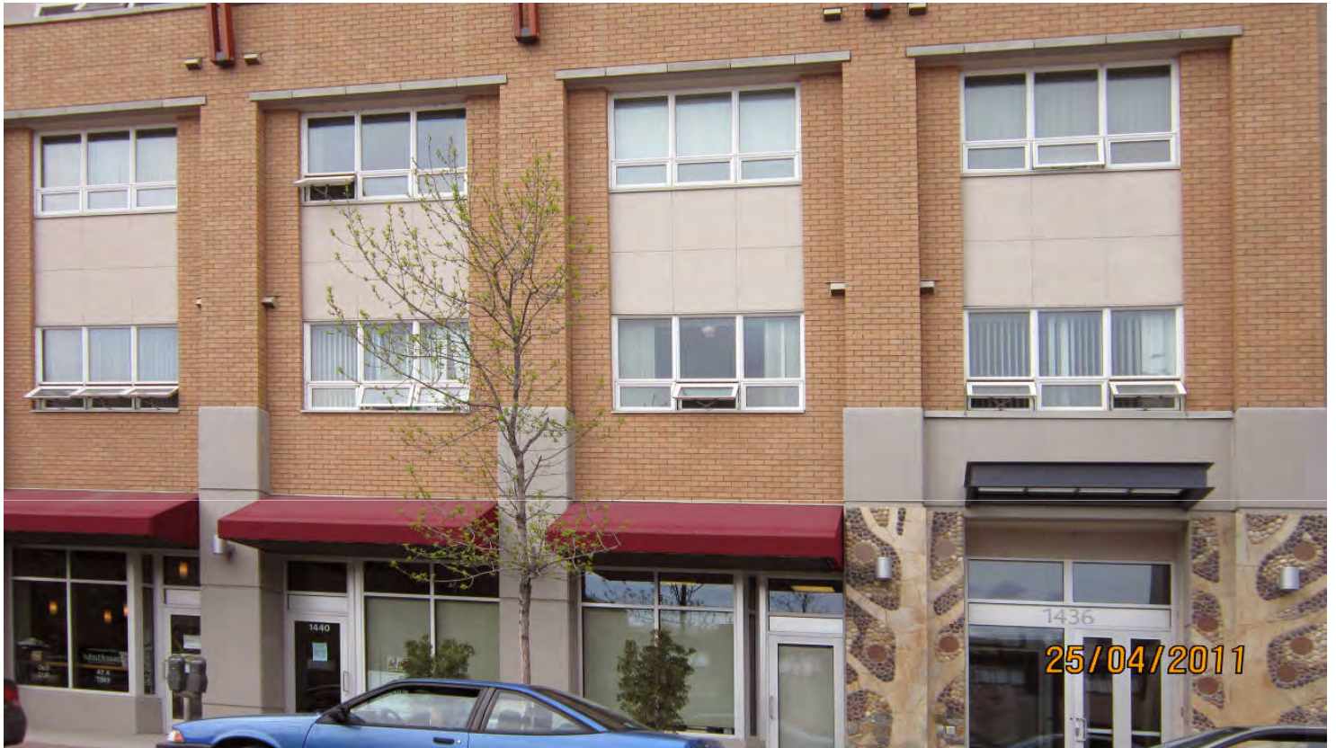
Pic. 133: Cardington Apartment, East Facade Source: Ulduz Maschaykh
