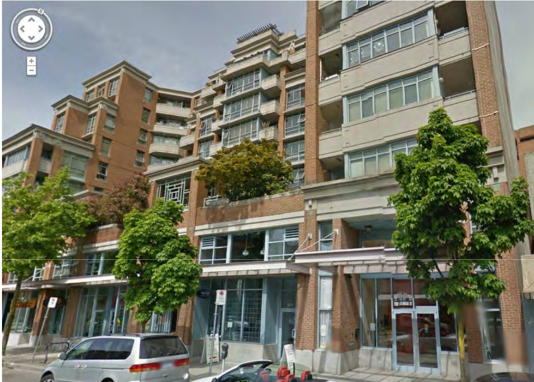
Pic. 59: Lore Kirll I, South Façade, Joe Wai, 2001 Source: Google Street View
