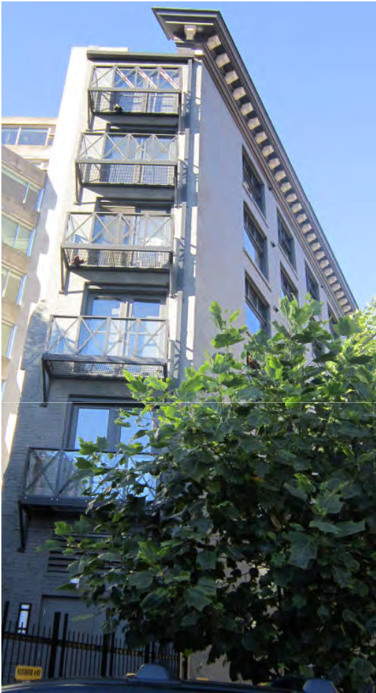
Pic. 77: Burns Block, South Elevation Source: Ulduz Maschaykh
