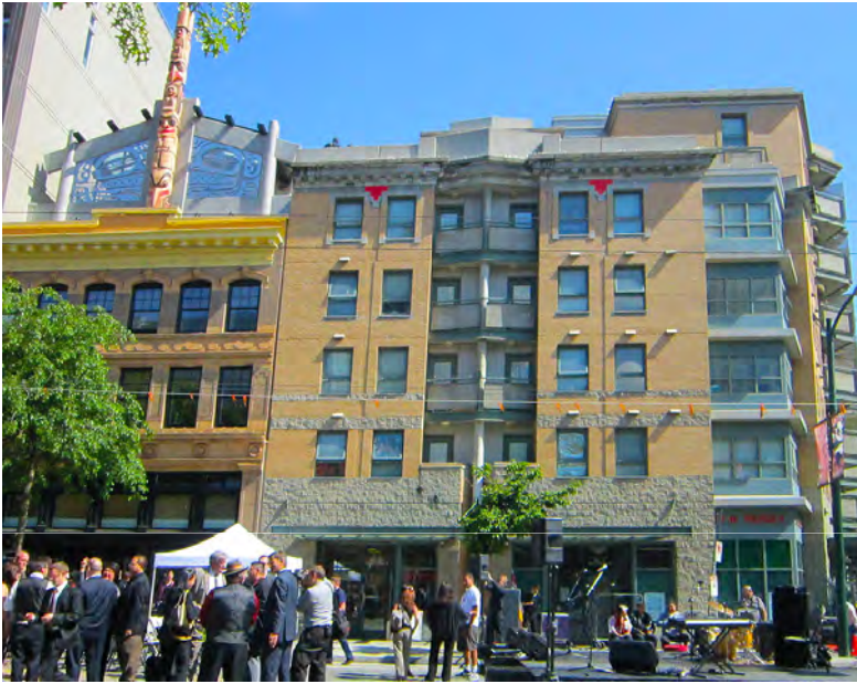
Pic. 89: Ian Leman Building, South Façade, Joe Wai, 2000 Source: Ulduz Maschaykh
