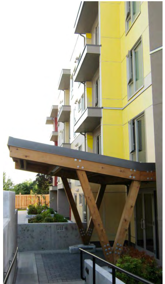
Pic. 53: Loreen Place , Main Entrance Door South Elevation Source: Ulduz Maschaykh
