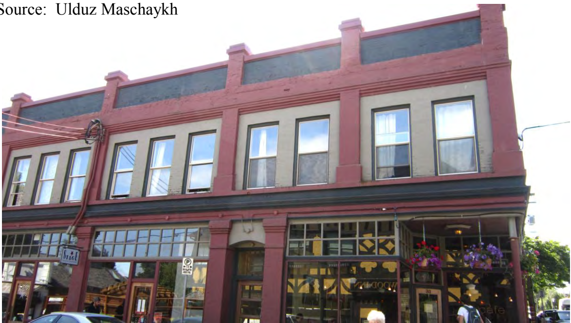
Pic. 35: North Façade depicting metal cornice, vertical pilasters and rectangular windows. Source: Ulduz Maschaykh
