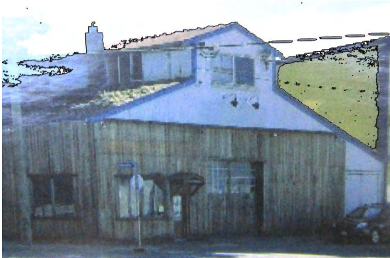
Pic. 47: Old Building 577 Pembroke, 1940. Source: Courtesy of Brad Shuya
