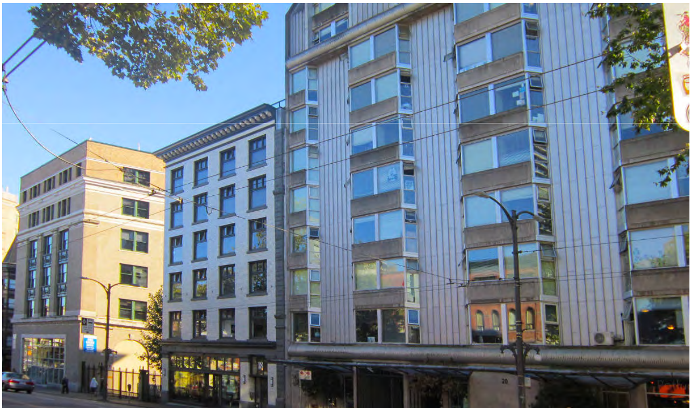
Pic. 76: Portland Hotel (right) and Burns Block (left) Source: Ulduz Maschaykh
