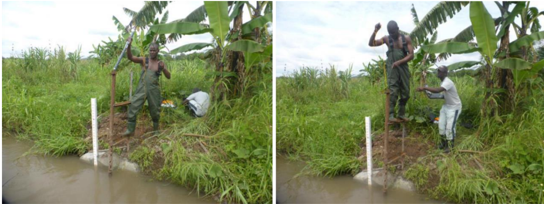
Fig. 3.3. Installation of the discharge gauge in the inland valley in Namulonge.
