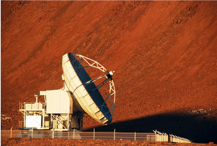
Figure 2.1: APEX Telescope at Llano de Chajnantor, Chile. The cabin behind the main dish, called the Nasmyth-B cabin, houses the new LAsMA receiver. This image has been taken from http://www.apex-telescope.org/ns/the-telescope/ .
