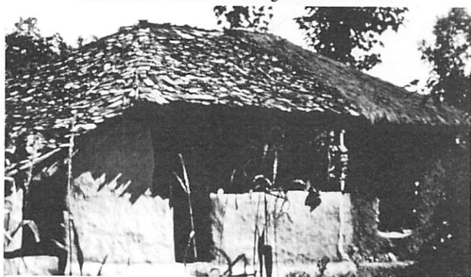
Below: Roof covered with shingles and rice straw.
