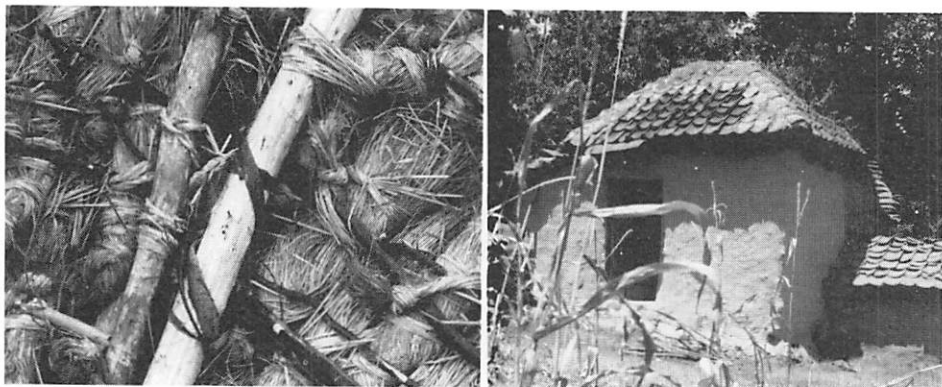
Above: Inside of a roof covered with rice straw.
