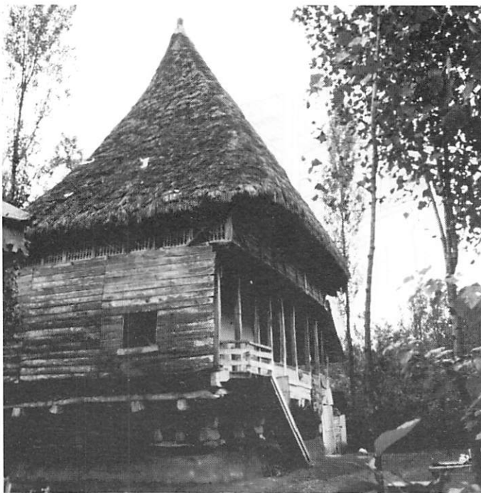
Foundations and base of a house in the Sefid Rud delta region. Substructure of stone and daub, pile of alternate logs and beams.
