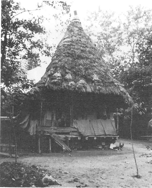
House of the Sefid Rud delta (note how it is raised above the ground)
