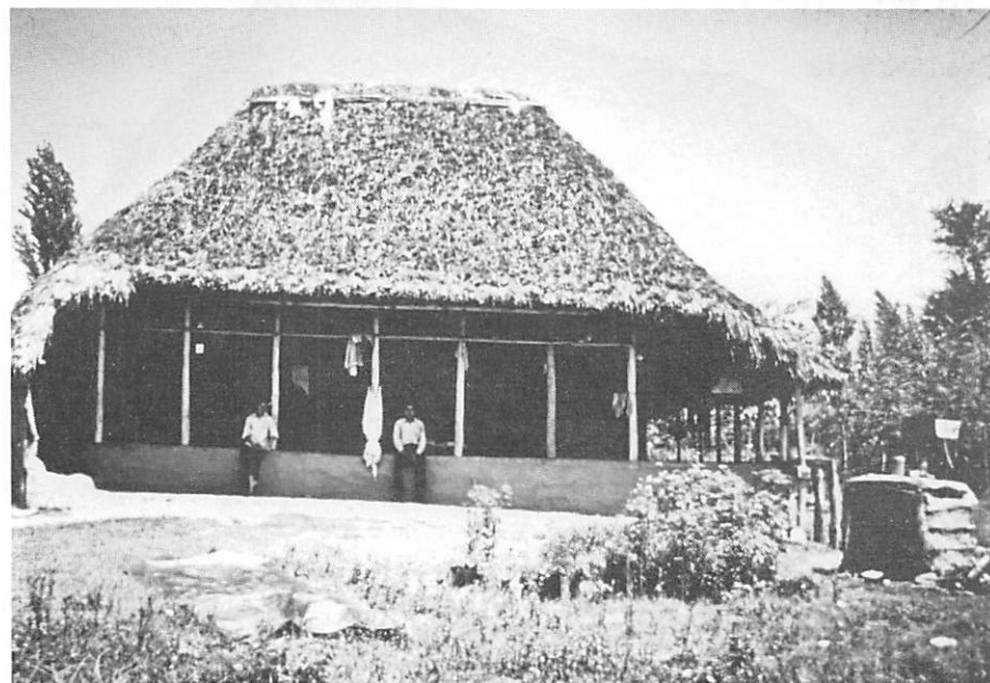
Above: house of the southern area of the Rašt district, with two talâr . Below: Single-storey house with the verandah extended down one side.
