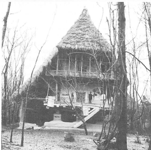
Two-storey houses with pointed roofs in the Sefid Rud delta. Note how they are raised above the ground.
