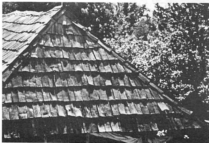
Roof covering of small boards (Tâleș piedmont)
