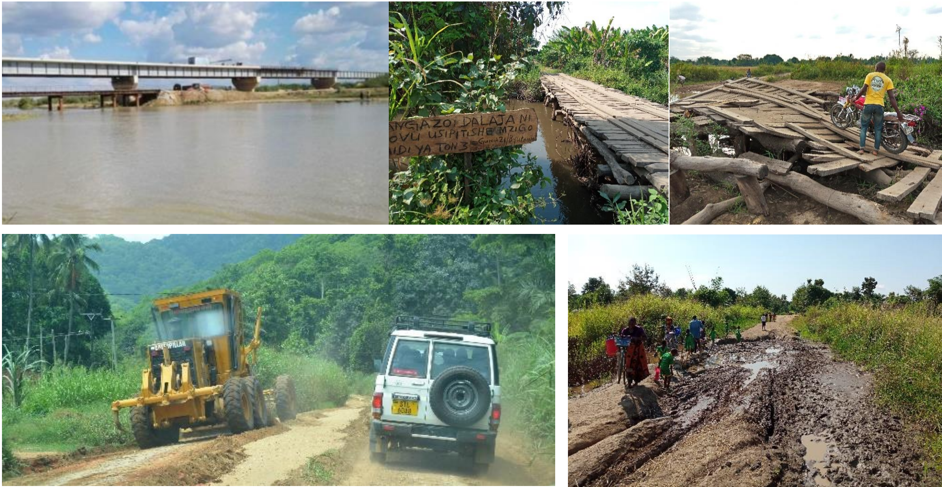
Figure 30: New Infrastructure in the Kilombero Valley
