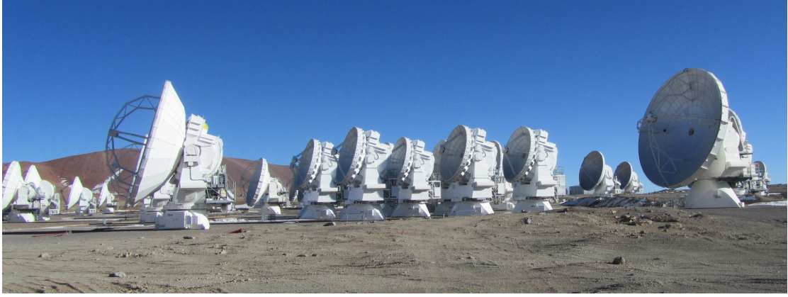
Figure 1.14: Some antennas of the Atacama Large Millimeter Array (ALMA) radio telescope in its compact configuration. Image credit: Manali Jeste.
