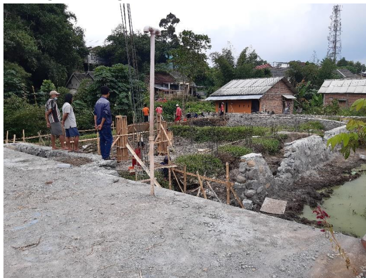
Figure 32 Bogeman Public Park Construction
