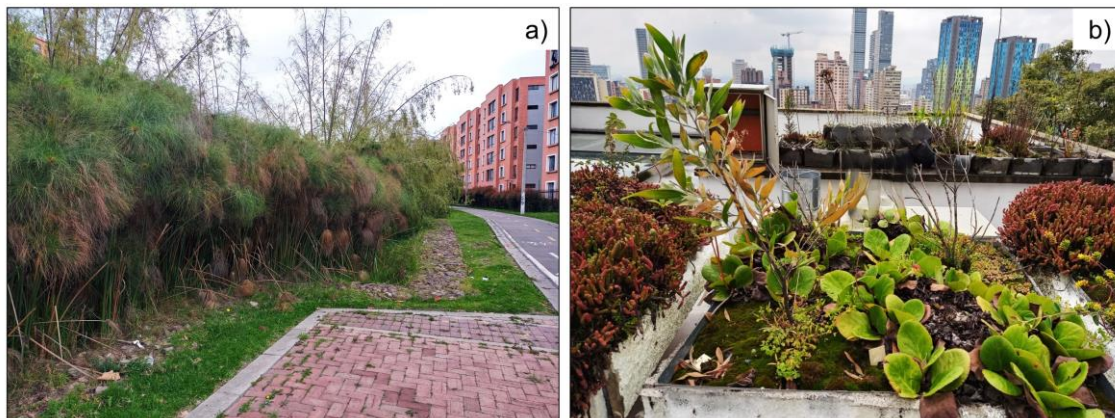
Figure 2.5 SUDS examples: a) bio-retention system in Soacha (a neighboring town of Bogotá) and b) prototype green roofs at the Universidad de los Andes, Bogotá
