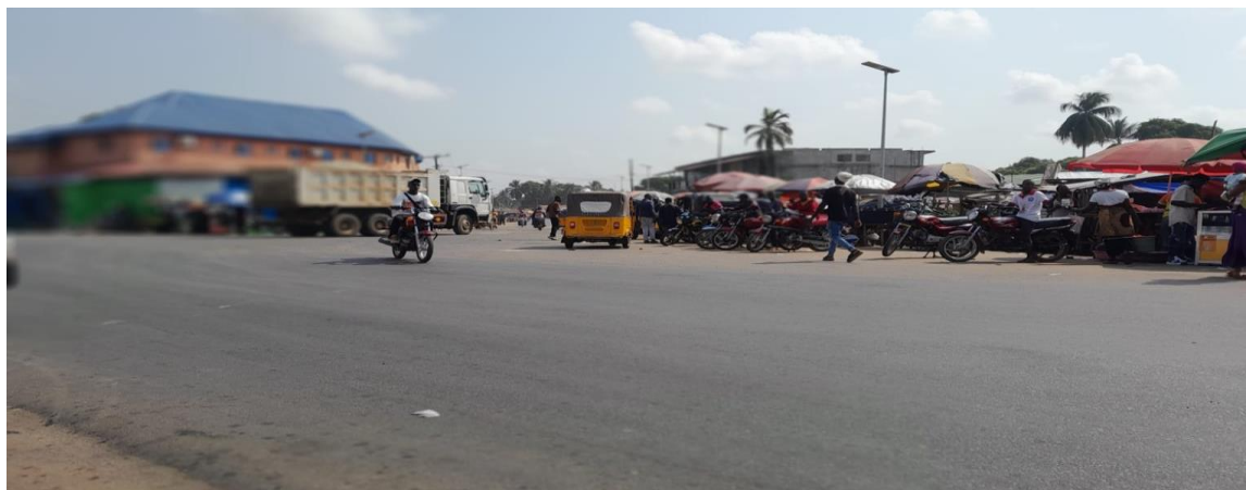
Figure 9: Solar-powered Street lights at Dry Rice Market, Barnesville Road (Author, 2023)
