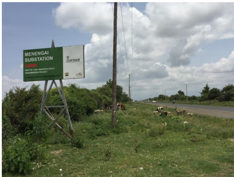
Figure 6: New power line for the Menengai geothermal project in Nakuru, Kenya
