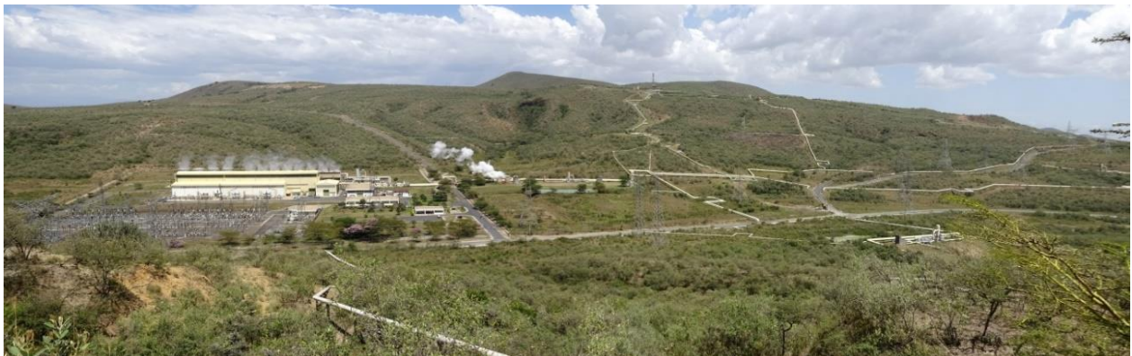
Figure 3: Geothermal power plant and infrastructure in Olkaria in Kenya
