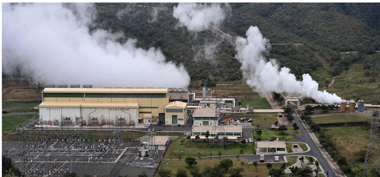
Figure 3: Aerial view of Olkaria II geothermal plants and SAGS
