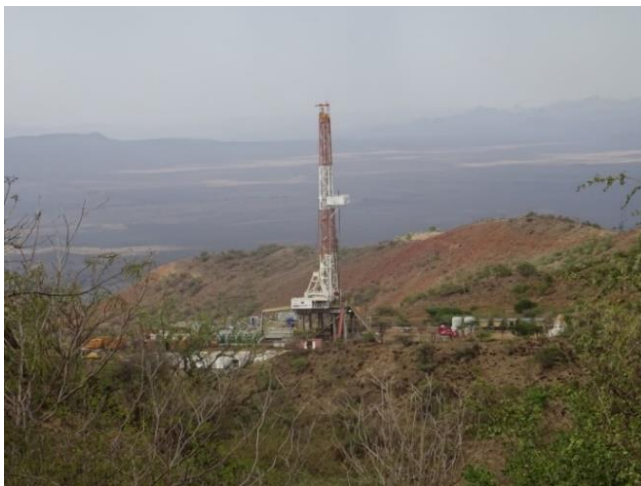
Figure 4: Drilling site in Baringo-Silali geothermal development project in Kenya
