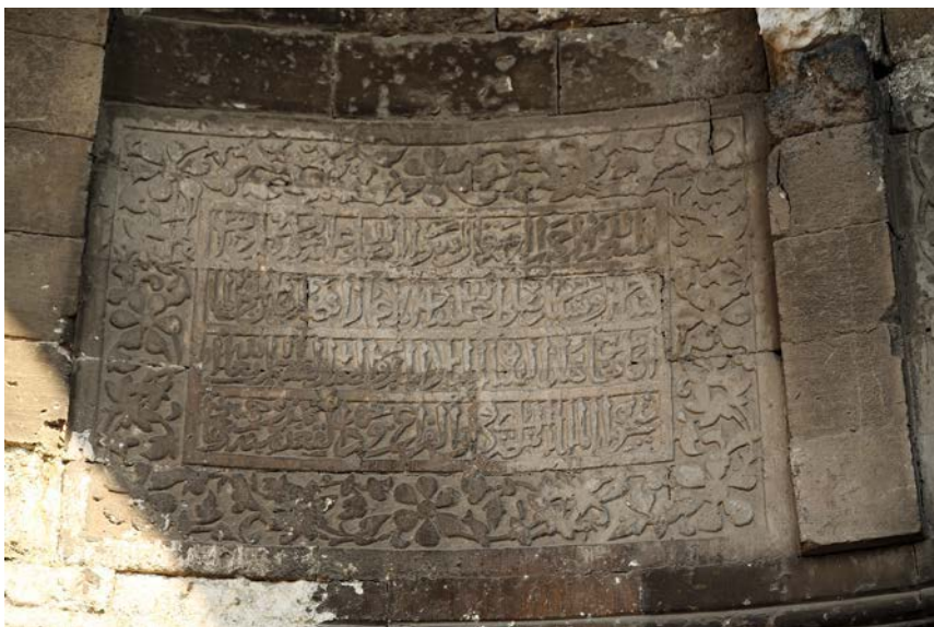
Fig. 20: The Sabīl of amir Shaykhū al-ʿUmārī al-Nāṣirī, 755/1354, entrance portal, foundation inscription panel over door.
