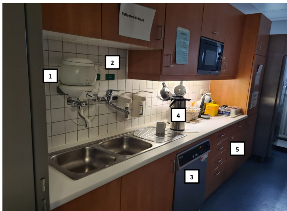
Figure 5. System diagram of a ward kitchen. 1: Decentral water heater. 2: PWC and PWH sampling point. 3: Dishwasher. 4: Coffee pot with pump. 5: Various coffeepots and teapots.
