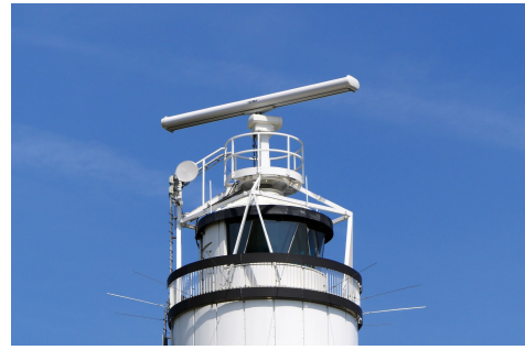
(b) maritime radar
