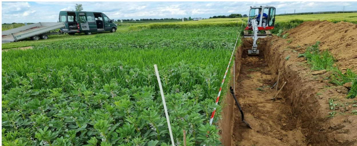
Figure S4.2: Trench across the experimental field measuring 1.5 m long and 1 m deep.
