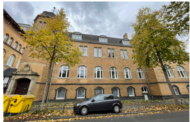
Figure 2. Street front of investigated building including 17 considered box-type windows in the basement, first, and second floor.
