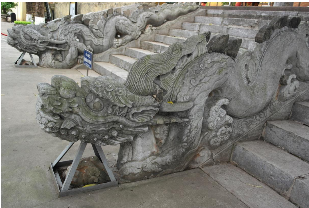
Fig. 81 Dragon steps to the Kính Thiên Palace (2018) with metallic support, 15th century, (Photo Courtesy of the Imperial Citadel of Thăng Long , photo taken by author)
