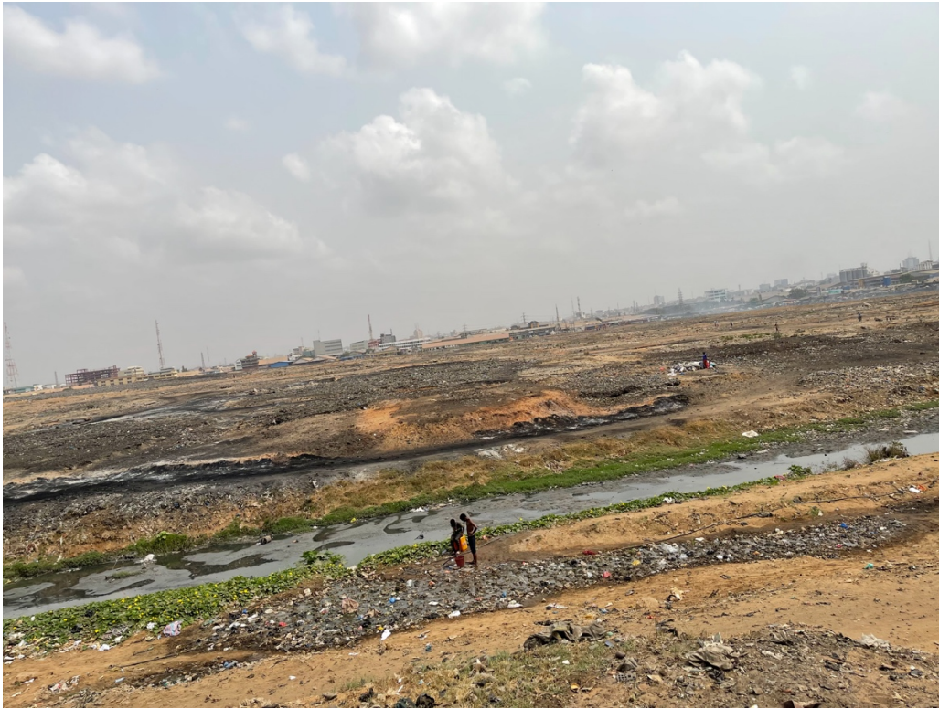
Figure 26. Aerial view of the Agbogbloshie site following the 2021 demolition. Source: Photograph by author, 2022.
