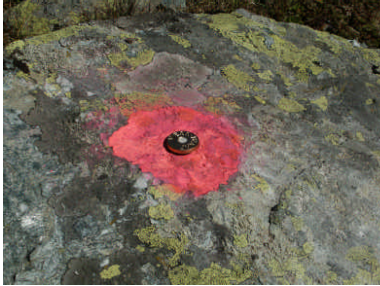
Figure 3.8: Steel dowels were drilled into the blocks for high-accuracy re-measurement. The thread, where the prism can directly be screwed into for the measurement, is protected by a plastic screw throughout the year.
