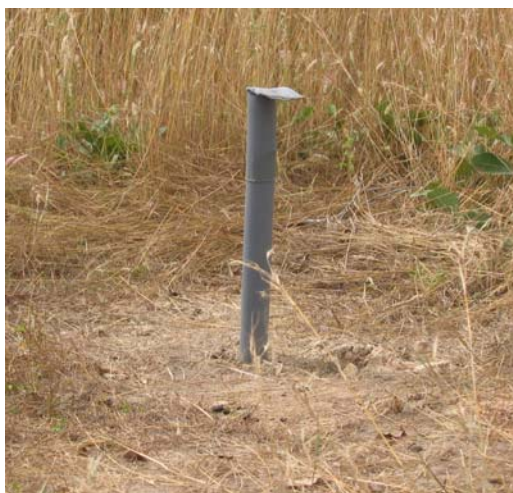
Figure 5.7: Piezometer with the pipe above the ground surface
