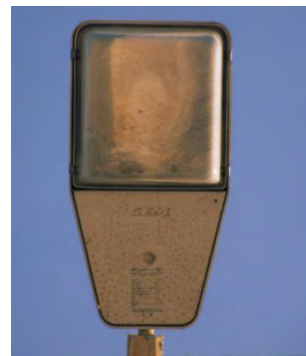
Figure 4.15: High Pressure Sodium Vapour (HPS) and car lights on coastal street (Section II). Mounting height of HPS lights: 10 m
