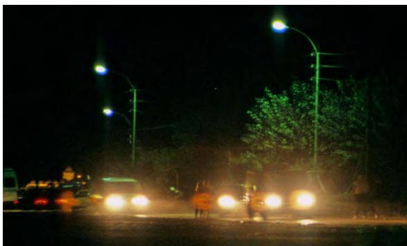
Figure 4.15: High Pressure Sodium Vapour (HPS) and car lights on coastal street (Section II). Mounting height of HPS lights: 10 m
