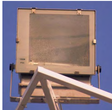
Figure 4.14: MH light in close proximity to a protected sea turtle nest (Section II). Mounting height: 8 m
