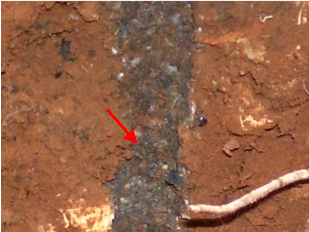
Figure 24. Walls of drainage tube lined with layer of propolis
