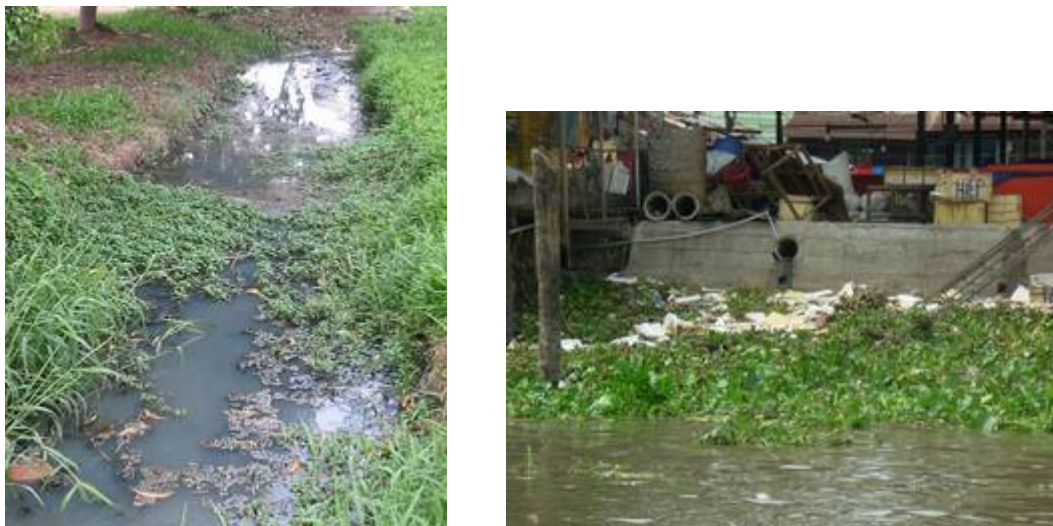
Figure 2-7: Sewers leading waste water untreated into the surface water of Can Tho Canal
