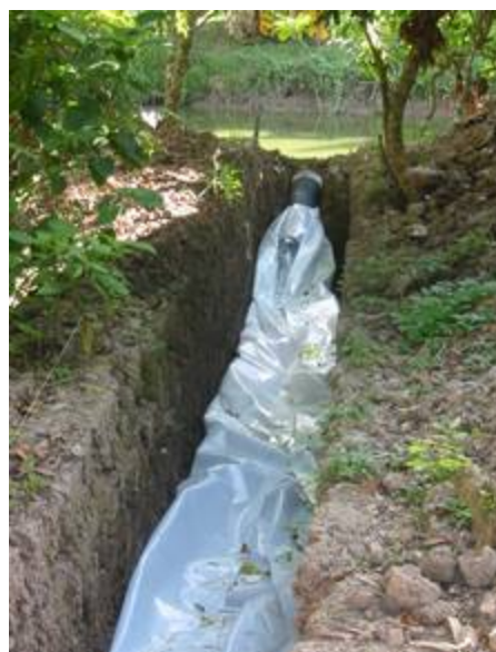
Figure 4-5: Plastic-tube reactor in the Mekong Delta during construction (outflow into the pond) and gas storage bag underneath a shelter
