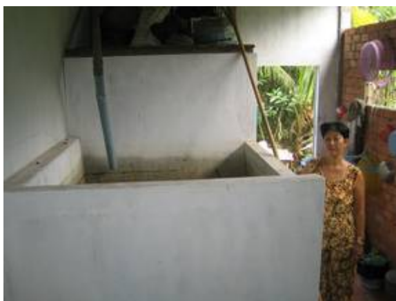
Figure 2-4: Rainwater storage at a rural household close to Can Tho
