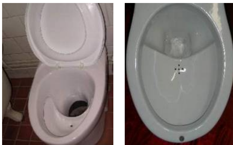
Figure 8-2: Low flush separation toilets, flushing for yellow water only (left), flushing for yellow and brown water (right picture)
