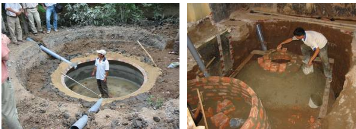
Figure 4-4: Fixed-dome reactors in Vietnam during construction
