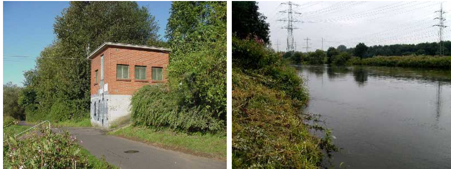
Figure 4.1: The left picture shows the gauging house of station Menden and the right picture the river Sieg on the underflow located near to the river Rhine (source of pictures: www.lds.nrw.de ).
