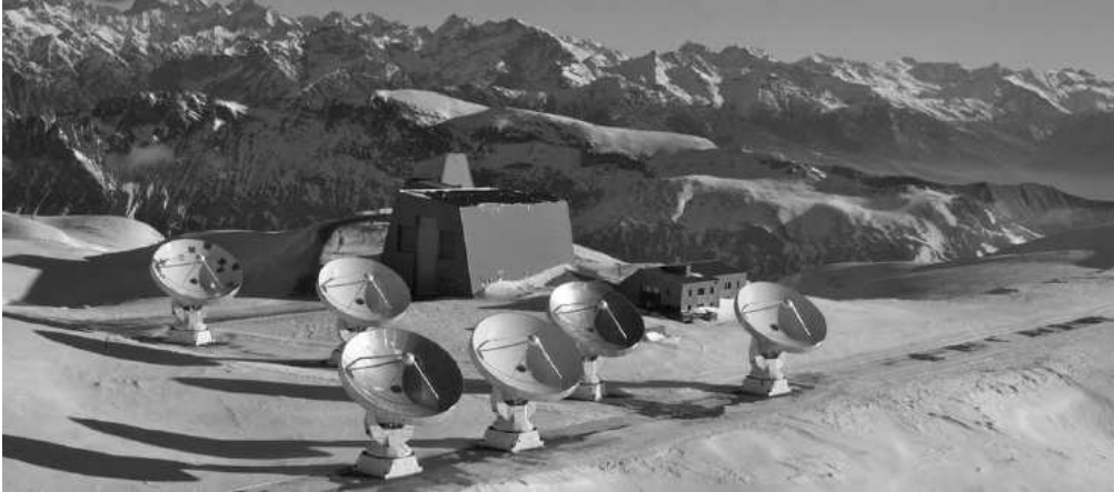
Figure 5.4: The IRAM Plateau de Bure interferometer in the French Hautes-Alpes, with six 15 m antennas (Image courtesy IRAM).
