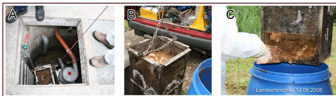
Figure 3.4. (A) Black water container of separated toilets, (B) the sieve collector of solid part from black water and (C) non-urine faecal matter (Fm) in Lambertsühle building of OtterWasser GmbH, Germany
